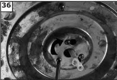
Loosen 2 screws with key slots and remove 1 screw without key slot. Place upper cover light kit over 2 screws and twist in direction of arrow to hold in place. Replace screw removed and tighten all 3 securely.
